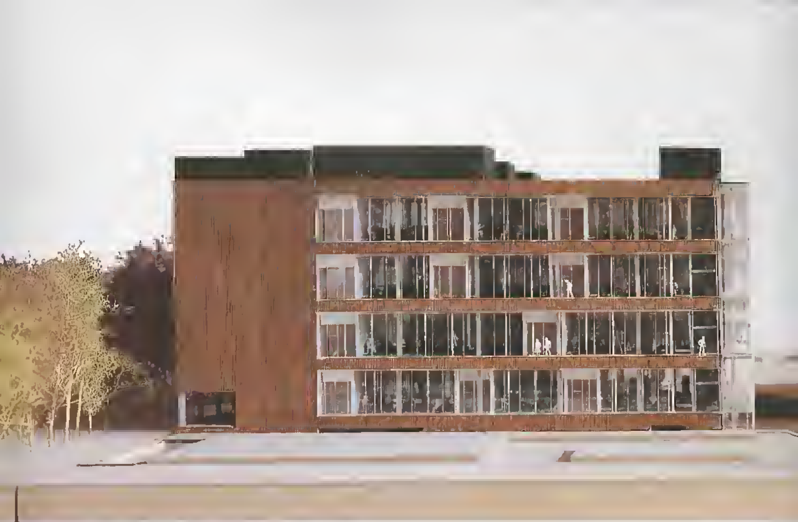
Vista de la fachada lateral (Sur-oeste) / View of side facade (Southwest)
